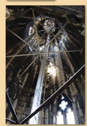
The spire is supported internally by a latticed steel framework. This modern construction method enabled the tower and spire to be built as if it were a small skyscraper, before, and independent of, the rest of the church.
